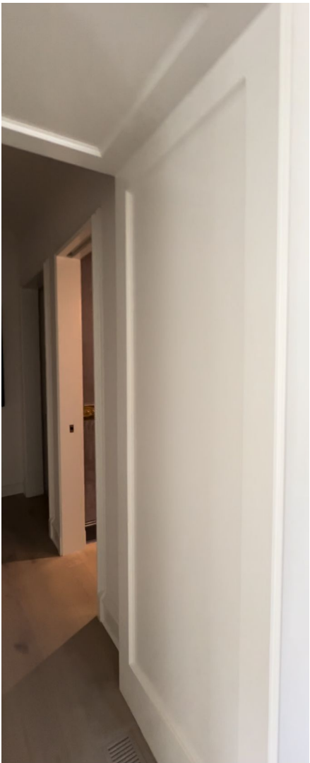
CASED OPENING W/ TOWERS PAINTED MILLWORK
