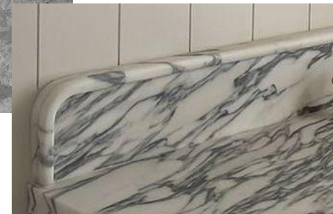
SLAB BULLNOSE - EDGE DETAIL
