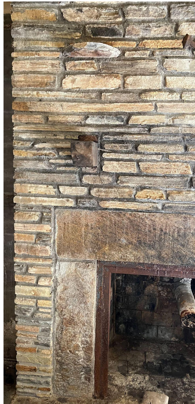
EXISTING FIREPLACE (CLOSE-UP)
