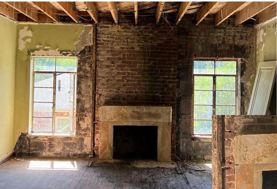
EXISTING FIREPLACE & FIREBOX - CLEAN SURROUND AND FIREBOX
